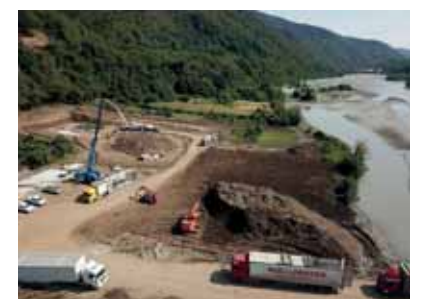
Construction of Namakhvani HPP. Source: lpress.ge
